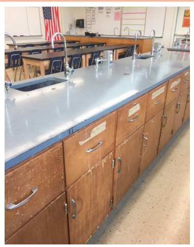
District 58’s middle school science labs are outdated, deteriorating and do not meet modern learning needs.
