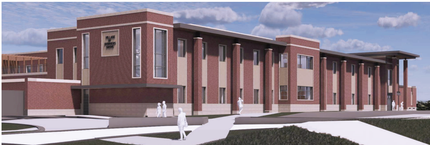
This rendering depicts the future Downers Grove Civic Center, a shared office space for District 58, the Village of Downers Grove and the Downers Grove Police Department.
