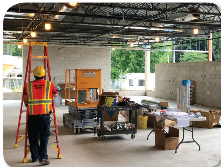
Crews spent this past summer building the Lester addition.
